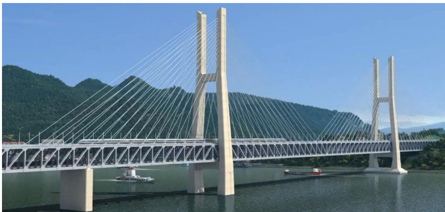
Fig. 4: The new Baishatuo Yangtze River Bridge
